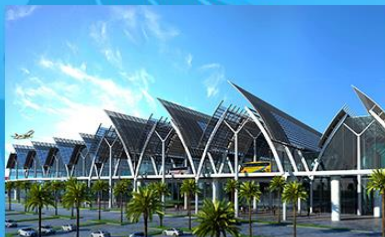
MACTAN-CEBU INTERNATIONAL AIRPORT (MCIA) PASSENGER TERMINAL BUILDING PROJECT
