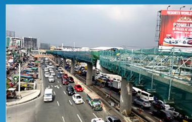
NAIA EXPRESSWAY (PHASE II) PROJECT
