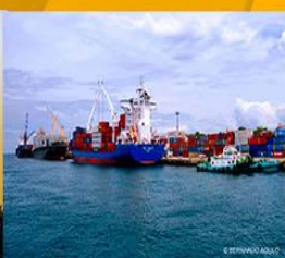
DAVAO SASA PORT MODERNIZATION PROJECT
