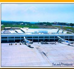
DAVAO AIRPORT OPERATIONS, MAINTENANCE & DEVELOPMENT PROJECT
